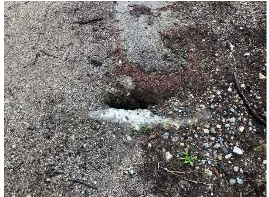
More damage to deck panels and ballast wall
