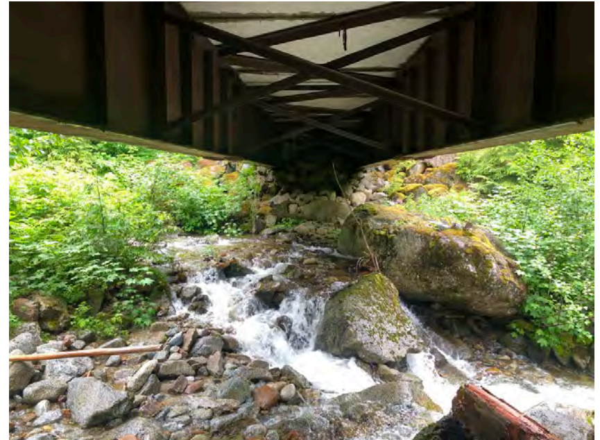
Left Bank Abutment when facing downstream
