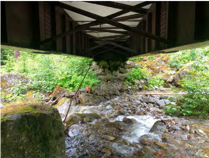
Right Bank Abutment when facing downstream
